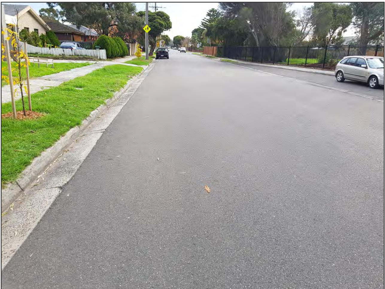
Figure 4 Coomoora Road, looking west along the site frontage
